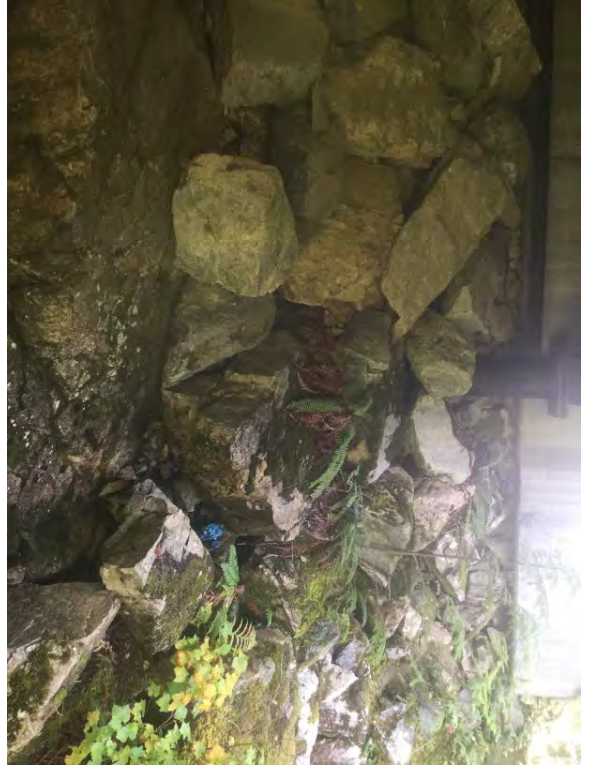
Right Bank Abutment when facing downstream
