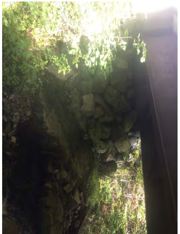
Right Bank Abutment when facing downstream
